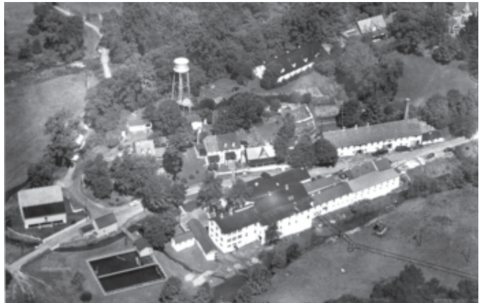
Now listed on the National Register of Historic Places, the Auburn Mills Historic District is shown here in 1958. This historic district is a combination of buildings that were either purchased or built by the Marshall family as part of Marshall Bros. Paper, the company that evolved into NVF. The Auburn Heights mansion is in the upper right corner. To the left of the mansion are the carriage house and Marshall Steam Museum, the home of the Friends of Auburn Heights Preserve and its collection of operating steam automobiles. The Auburn Mill, now owned by Delaware State Parks, is across the bottom, with the Red Clay Creek alongside.
